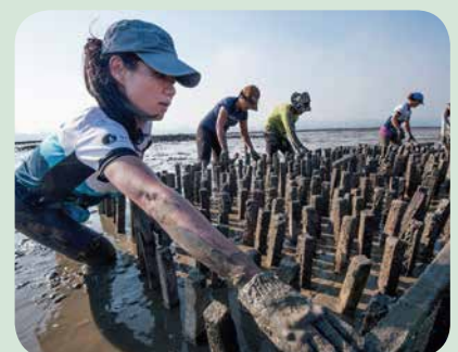
Building pilot reefs in Lau Fau Shan, Deep Bay. © Kyle Obermann
